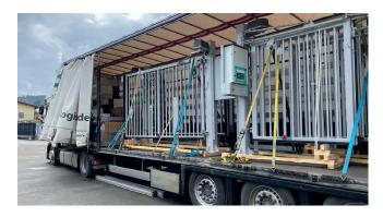
This means a drastic reduction in assembly times. The time for the required forklift or crane is also reduced. In addition, templates for the base plates are available from ZABAG in advance. This enables the installer to set the anchor bolts before delivery.
